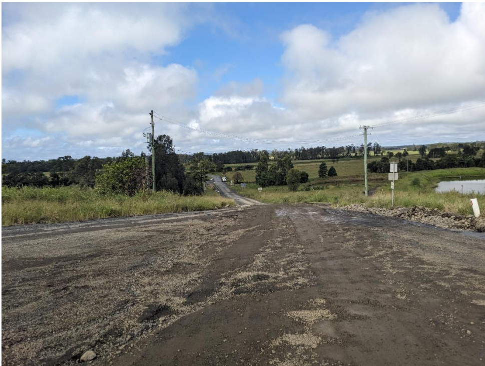
Site entrance adjacent to the site office, requiring some reshaping to ensure dirty water enters the sediment basin to the right
